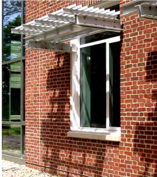
Sunshade, south-facing window, North Academic Building
